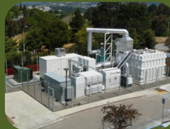
1.4 MW DFC1500® • Utilizes one module • Adequate to power 1,400 homes
