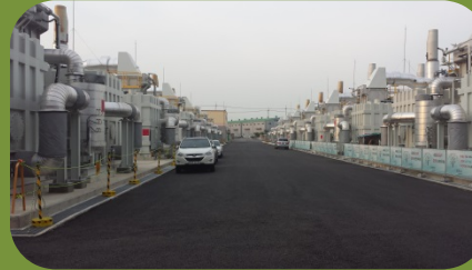
59MW fuel cell park • Utilizes 21 DFC3000 plants
