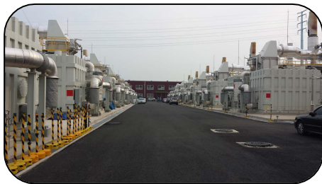
59 MW fuel cell park
