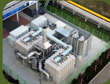
2.8 MW DFC3000® • Utilizes two modules • Adequate to power 2,800 homes
