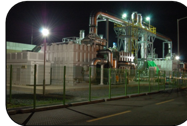
5.6 MW fuel cell park
