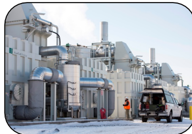
14.9 MW fuel cell park
